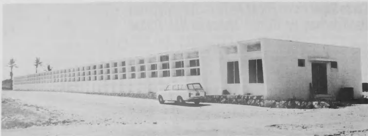
The former High School now converted into a one-story Community Services facilities.
